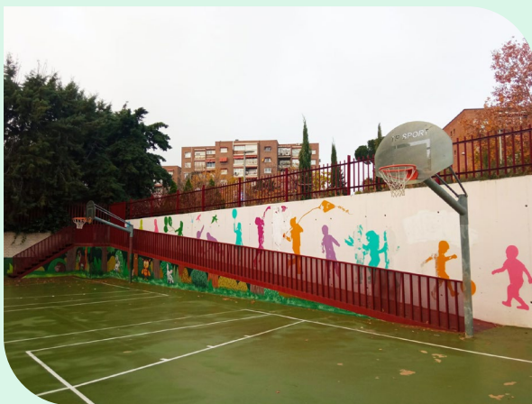
Picture 3: The ramp which I use to access to my school © Lucia
